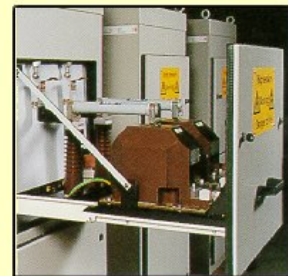
Draw out voltage transformer with primary fuse
